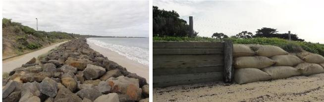
An exposed seawall will change the natural aesthetics of the beach and coastline. Exposed seawalls are typically used only as a last line of defence to protect critical assets (a last access road or other critical infrastructure) and in urbanised foreshore environments.
