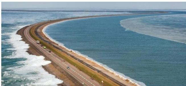
**Dykes and levees** take the form of elevated mounds or walls that can be made of earth, rock, concrete, geo-fabric bags or other materials.
