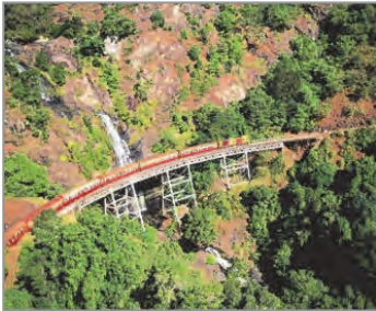
PICTURESQUE RAIL BRIDGE OVER STONE CREEK, KURANDA SCENIC RAILWAY (PHOTO: WTMA)
