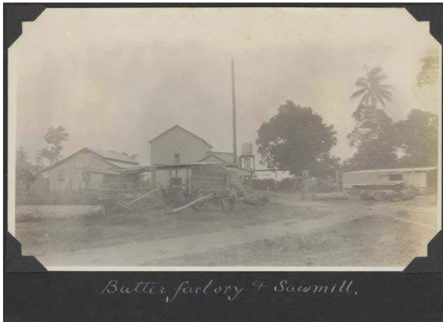
Figure 34: Butter factory and sawmill at Daintree (Source: National Library of Australia).
