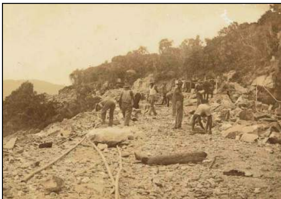
Figure 26: Building the Cairns- Port Douglas Highway. (Source: Billi Noli).
