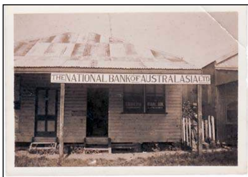
Figure 31: The first national bank of Australasia building in Mossman. (Source: National Australia Bank Archives).
